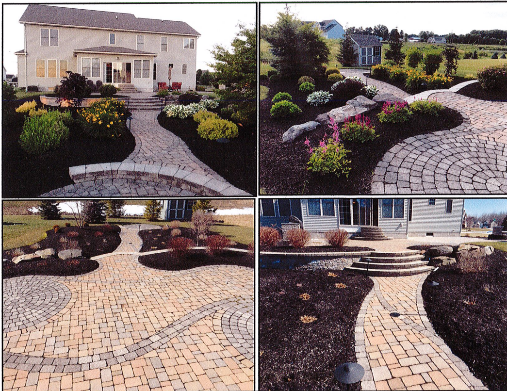
Photographs showing elevations and features of the existing hardscape and landscape.
